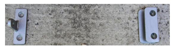
5. Remove the brackets and drill out the 4 holes where you have marked it.
