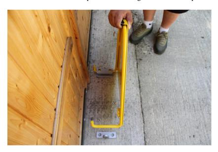
4. Mark the 4 holes with a pencil on both brackets on the surface.
