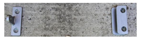
Remove the brackets and drill out the 4 holes where you have marked it.
