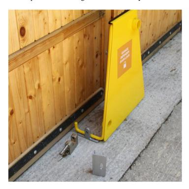
Put the security plate over the bracket to secure the frame.
