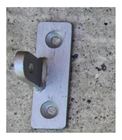
Now slide the plate with the legs over the security bolts and brackets.
