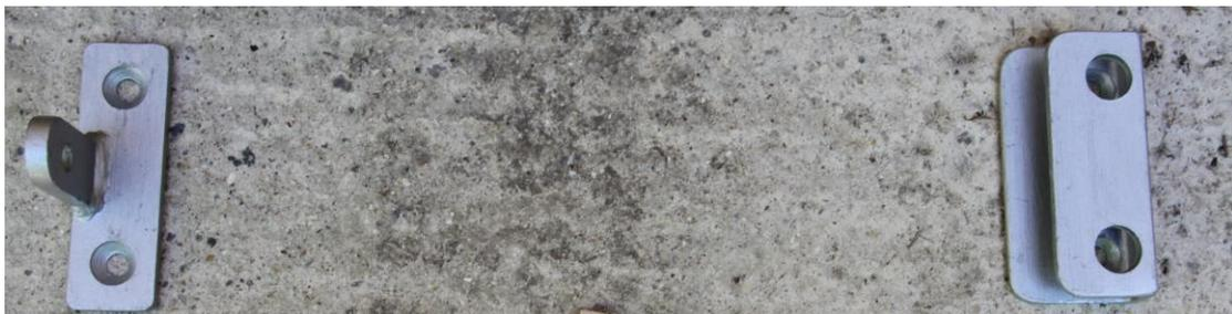
Remove the brackets and drill out the 4 holes where you have marked it.
