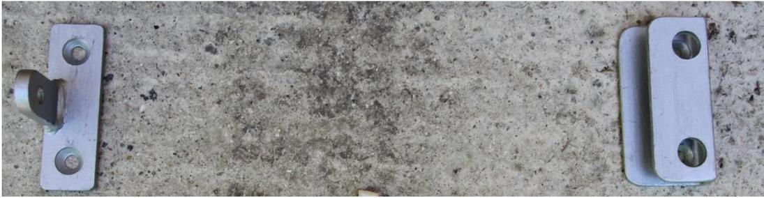
*4. Mark the 4 holes with a pencil on both brackets on the surface.*
