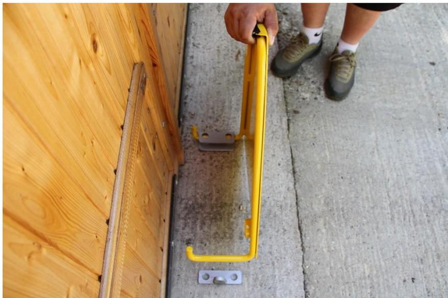
*3. Slide out the complete unit leaving the brackets in place.*
