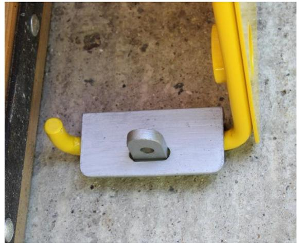
*9. Put the security plate over the bracket to secure the frame.*
