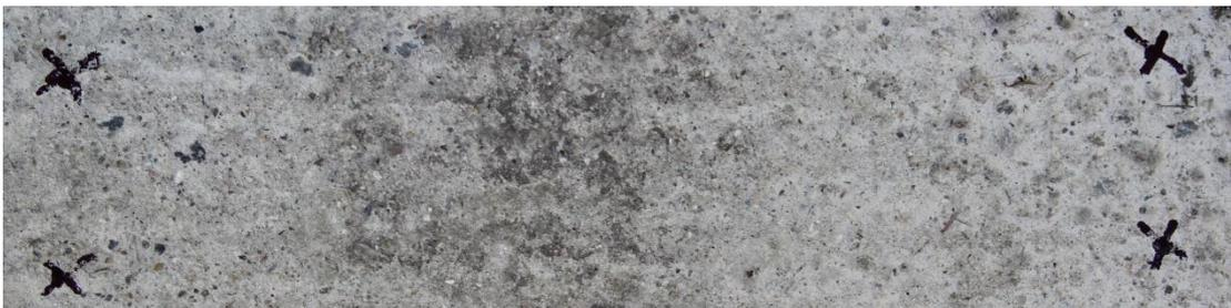
*5. Remove the brackets and drill out the 4 holes where you have marked it.*
